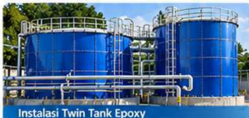
Instalasi Twin Tank Epoxy
