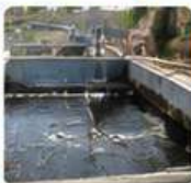
WWTP / IPAL Wastewater Treatment Plant
