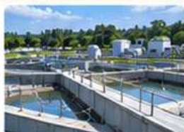
WTP / IPA Water Treatment Plant
