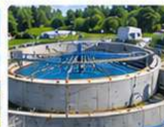
Municipal Water Treatment
