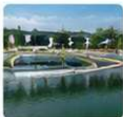
WTP / IPA Water Treatment Plant
