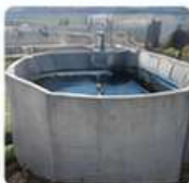
STP Sewage Treatment Plant
